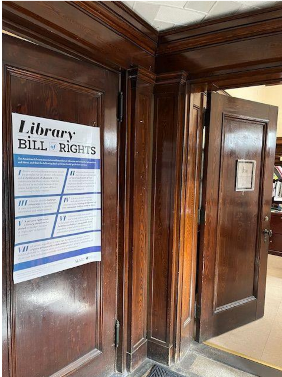
Original wood trim and wood doors with a corner of the Guastavino tiles in front entryway
