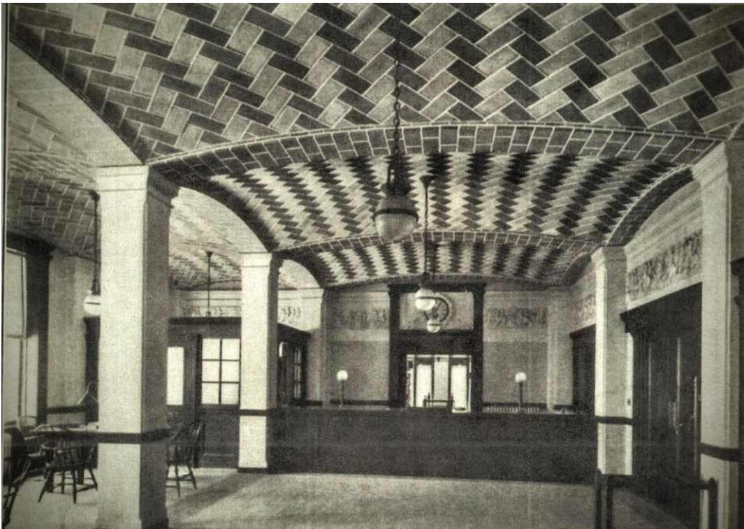
The Circulation Desk of 1903 remains the focal point of service
