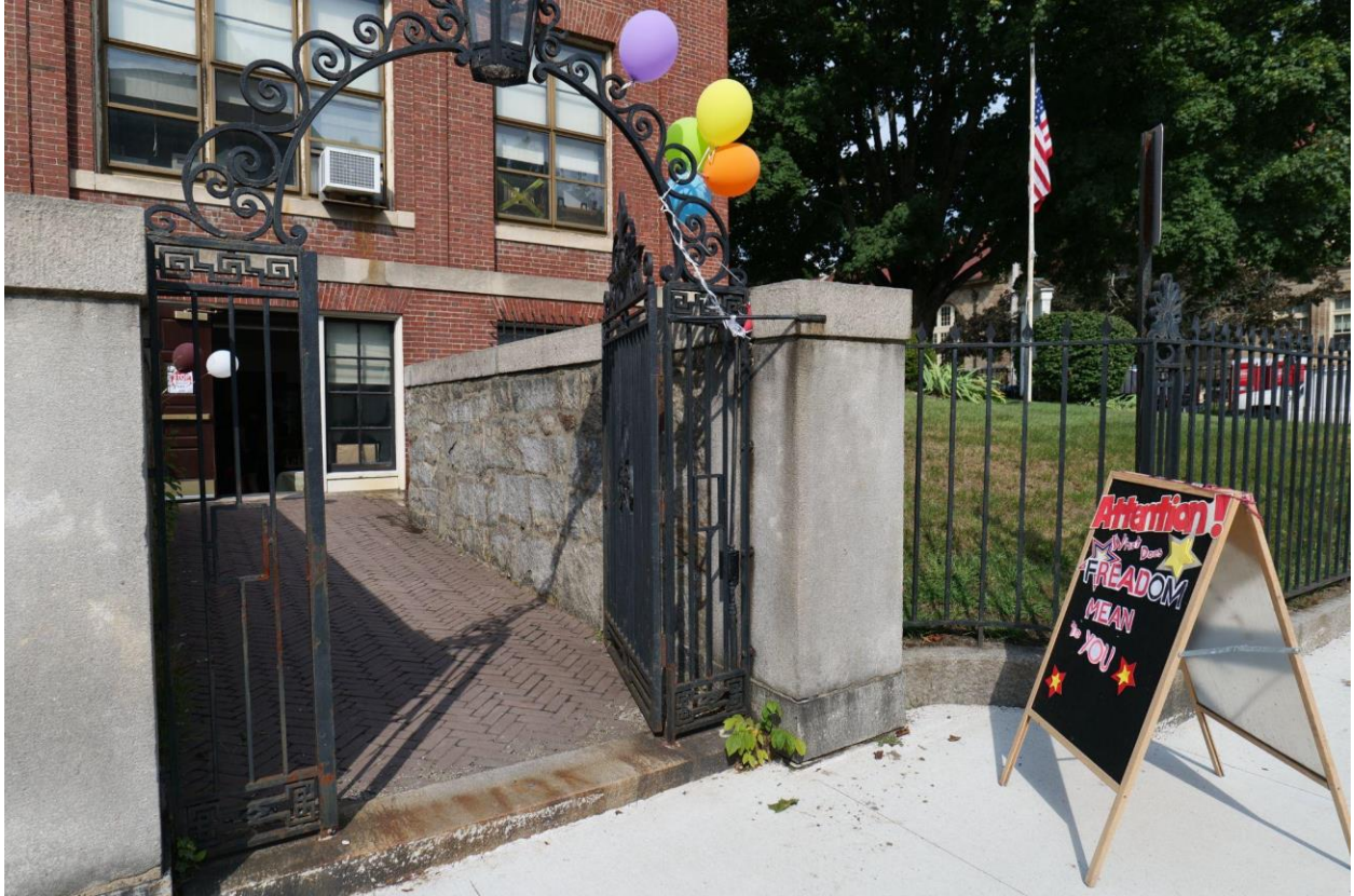
Side door on Church St, usually an emergency exit only, leading from the Community Room. During the Friends of the Library Book Sale, it is a non-ADA-compatible entrance. Brick walkway was reset in 2016. (It wasn't just repointed, they replaced all the bricks)
